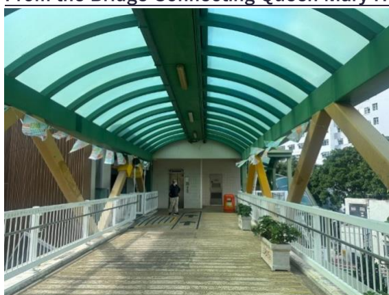
1. Walk across the bridge towards Sassoon Road.
